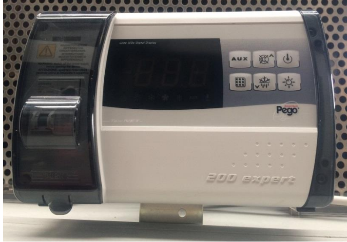
Picture 2 - Control panel of the refrigeration unit
